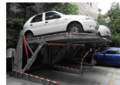
Postposition cantilever sort Rear cantilever structure, hydraulic drive.
